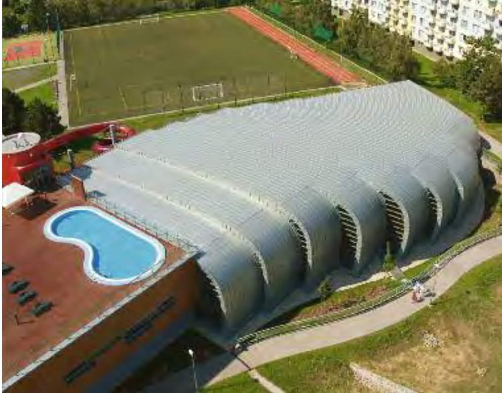
Metal standing seam roof over aqua-park
