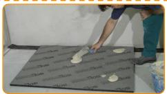
Apply the glue on the panel by spreading it Apply the panel on the wall by forcing with on dots.
