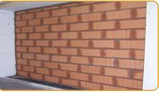
Build up the wall by caring to joint the blocks Apply in the first wall a layer of row mortar with mortar on both vertical and horizontal ioints.
