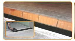
Lay the under wall strip in the dry floor before to build the wall.
