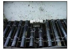
Temporary metal pipe lay-over method zip-tied in place
